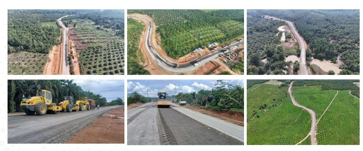
Upgrade of the coal hauling road using CTRB (Cement Treated Recycling Base) to improve road durability and maintain hauling truck performance in support of production
